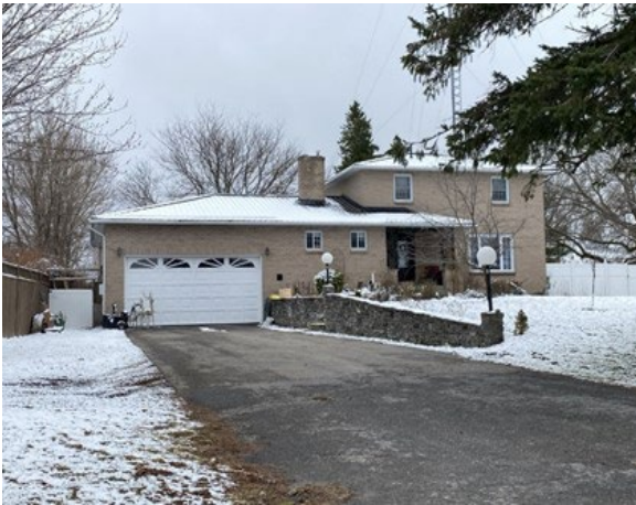
Photo 3 Representative mid-20 th century split-level residence at 2803 Concession 2, looking southeast
