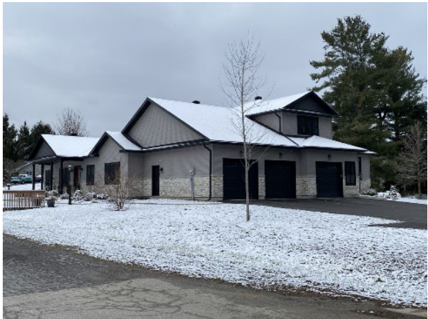
Photo 4 Representative photo of a new build farmhouse located at 2863 Concession 2
